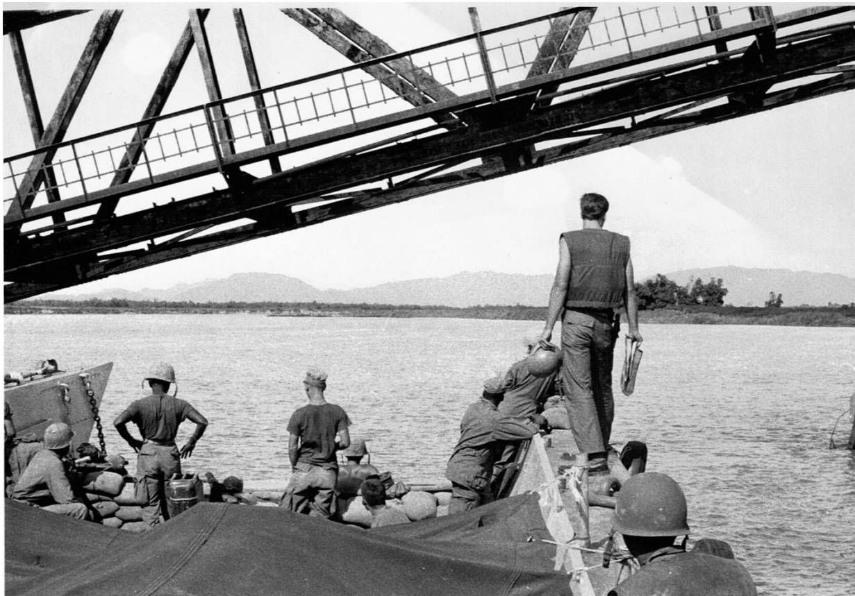
Figure 4 - Picking our way under a downed span of the bridge, August 18, 1966.
